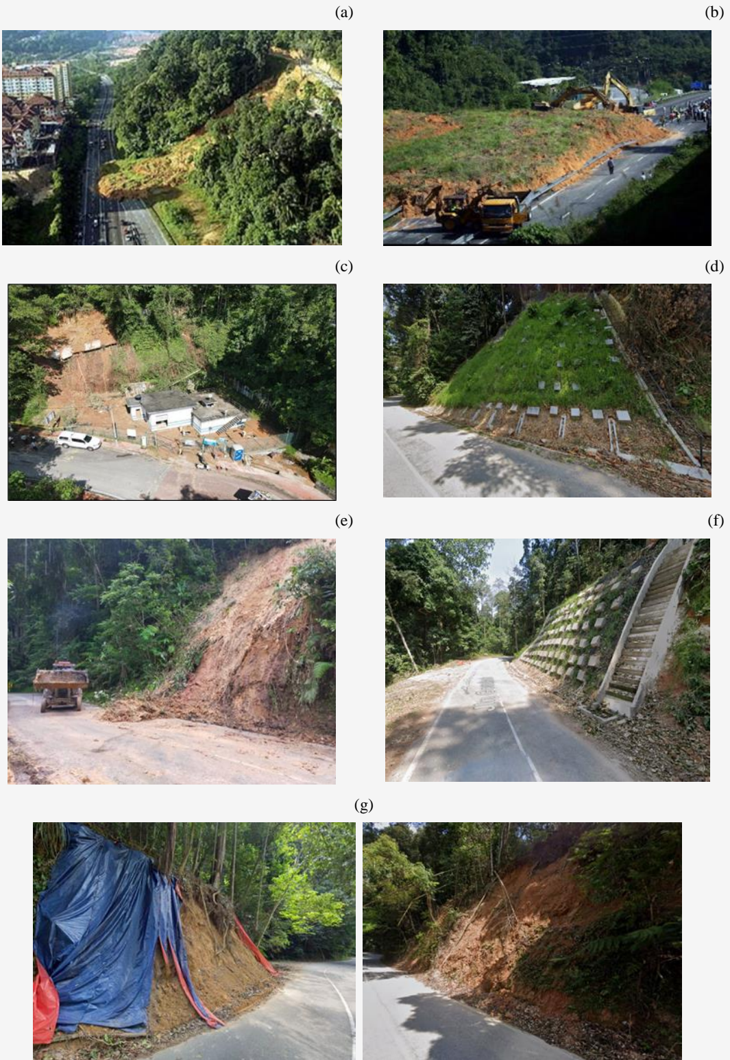
Figure 6: Photographs of landslide inventory locations obtained from archival documents within the MPS purview: (a) Taman Amansiara, Selayang; (b) Jalan Selayang-Templer in 2009; (c) Taman Selayang Permata in 2023; (d, e, f, g) show landslides occurring at various locations along Jalan Gombak Lama – Genting Sempah, some of which have already been repaired
